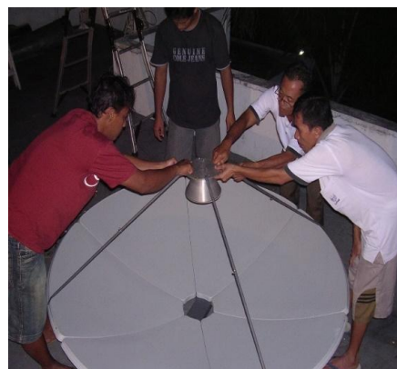
Figure 7. Install Feed Horn on Parabola
