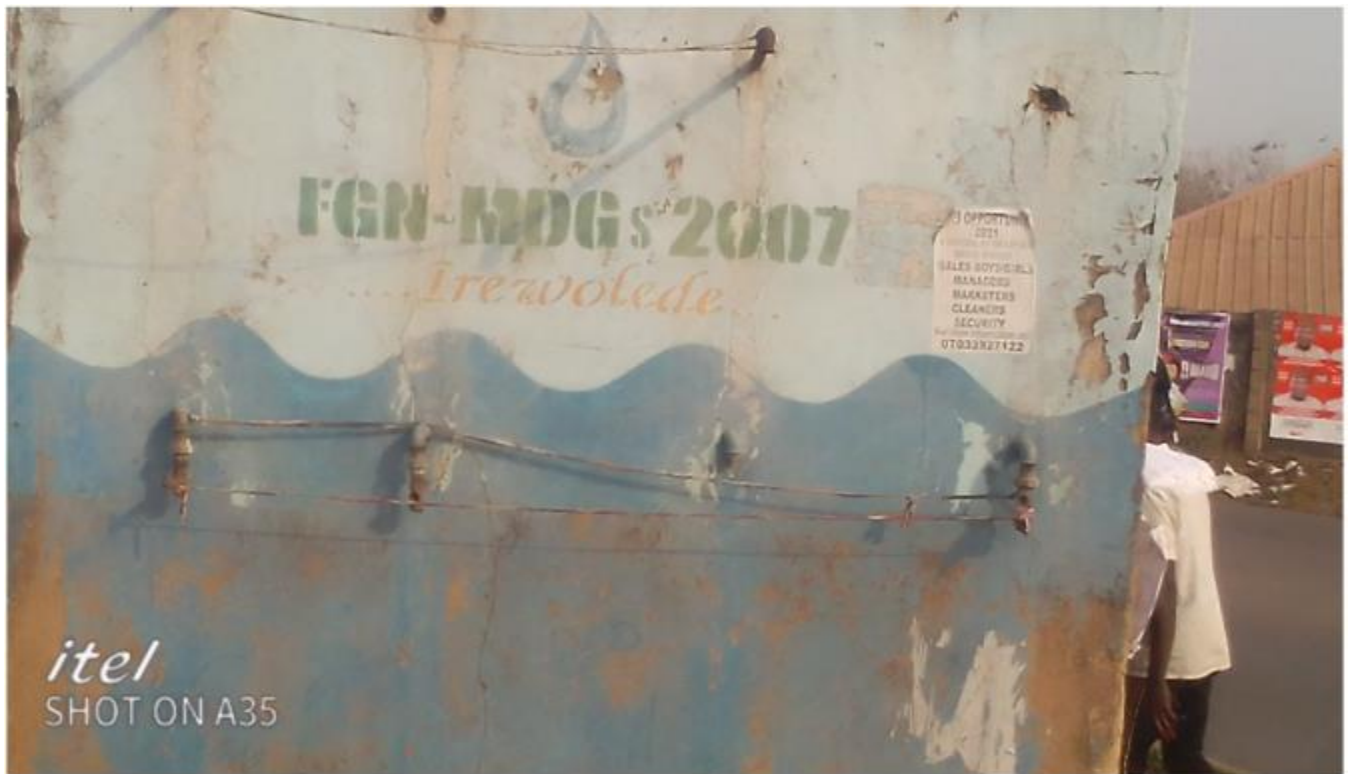
Fig 4. Abandoned MDGs water project, Oke-Ori Omi, Ado Ekiti.
