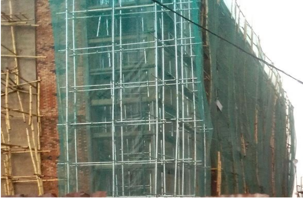
Fig 6(a). Insecticide Mosquito nets been used as fence at construction site in Ado Ekiti
