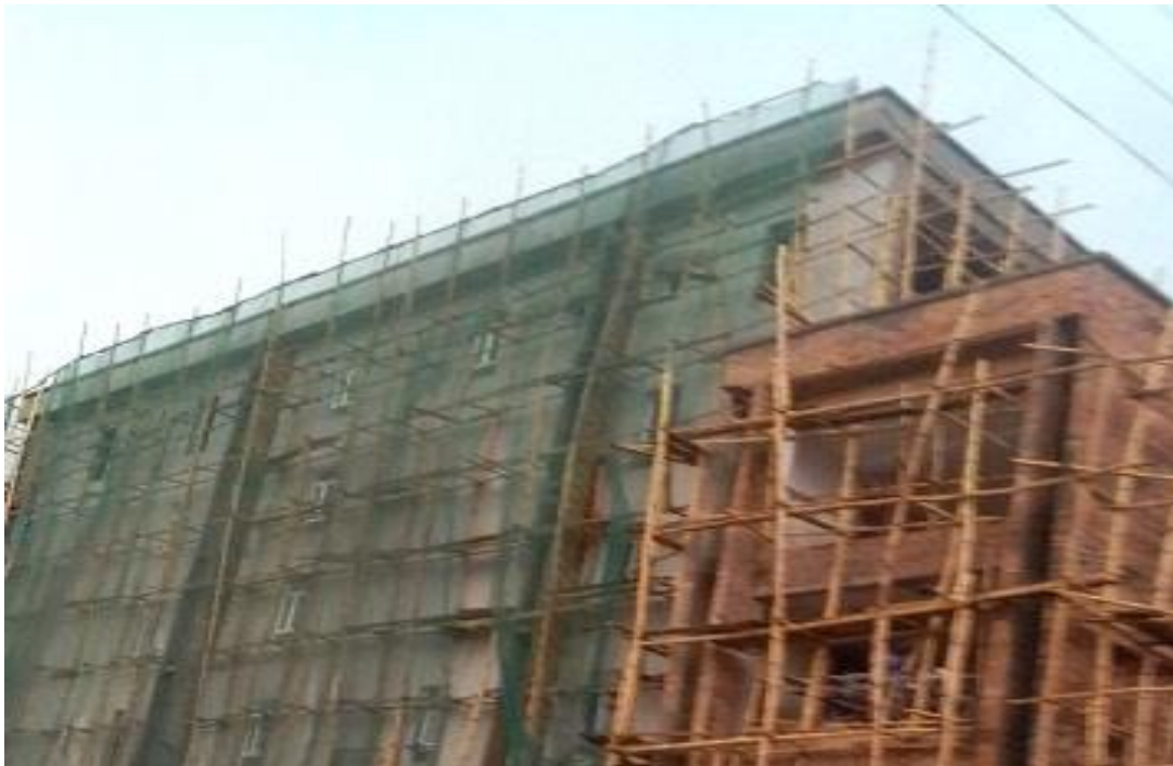
Fig 6 (b). Insecticide Mosquito nets been used as fence at construction site in Ado Ekiti
