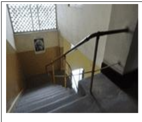
Figure 7 (left) is a photograph showing added balustrade to staircase (element value) and figure 8 (right) is a photograph which modified window whereby hardwood louvers were replaced with glass shutter and steel bars added to take care issue of security. (element value)
