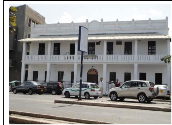
Figure 5 (left) is a photograph of a White Fathers building before alteration while figure 6 (right) is a photograph of a White Fathers building after the addition of columns (which created veranda at ground floor and balcony at the upper floor), decorated balustrades and a gentle slope pitched roof for balcony at the first floor
