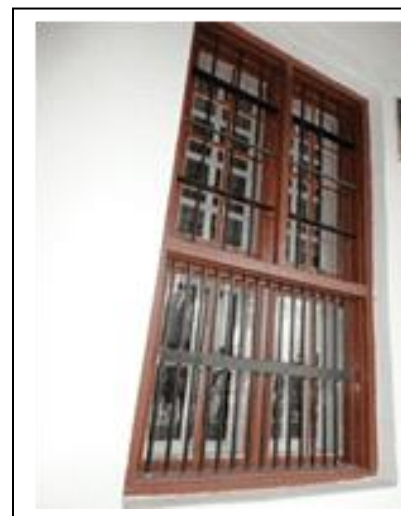
Figure 7 (left) is a photograph showing added balustrade to staircase (element value) and figure 8 (right) is a photograph which modified window whereby hardwood louvers were replaced with glass shutter and steel bars added to take care issue of security. (element value)
