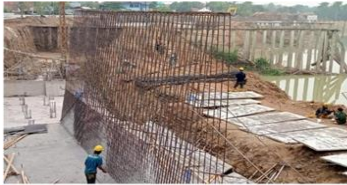
River Bank Protection Development Process in Pabedilan Village, Cisanggarung River Area, Cirebon Regency, West Java Province
